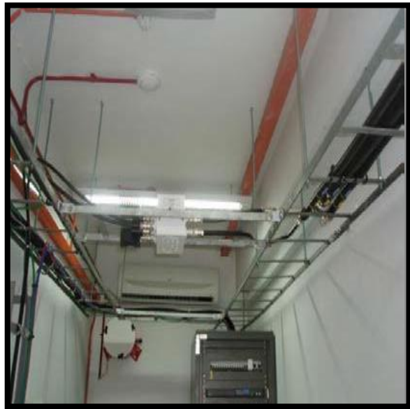
CABIN INTERNAL CABLE LADDER
