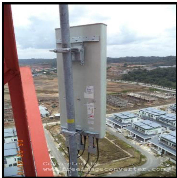
ZTE ANTENNA INSTALLATION
