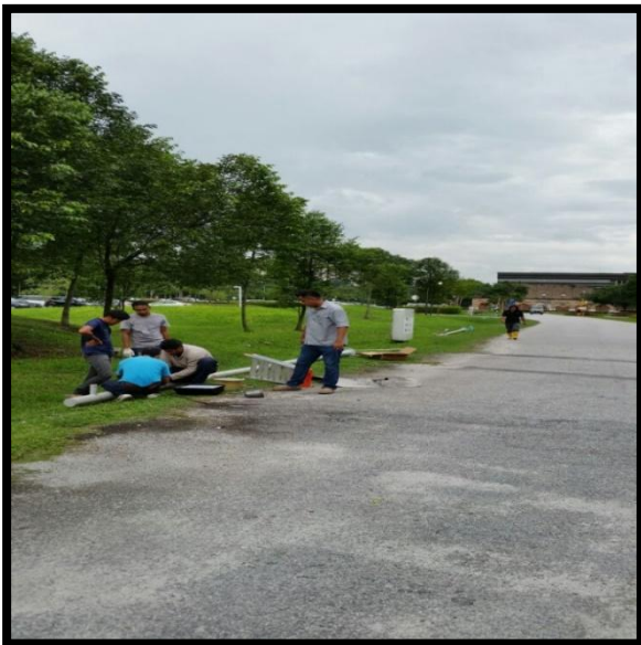
SENTUL RAYA – INSTALLATION OF 250W FLOODLIGHT POLE COMPOUND LIGHT
