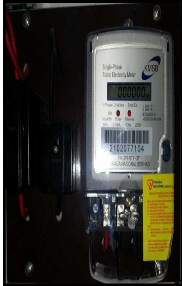
METER PANEL INSTALLATION
