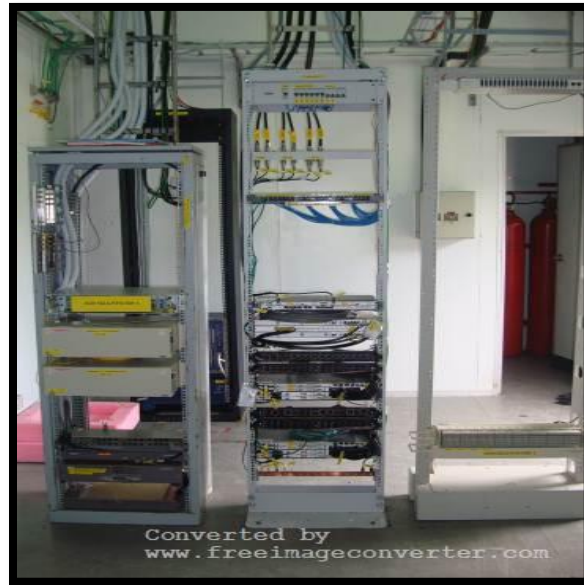
LINK HUAWEI 19 INCH RACK INSTALLTION
