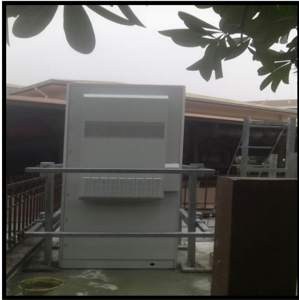
Installation T5 Cabinet C/W Lock Bar
