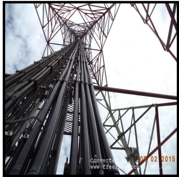
ZTE FEEDER 15/8 INSTALLATION
