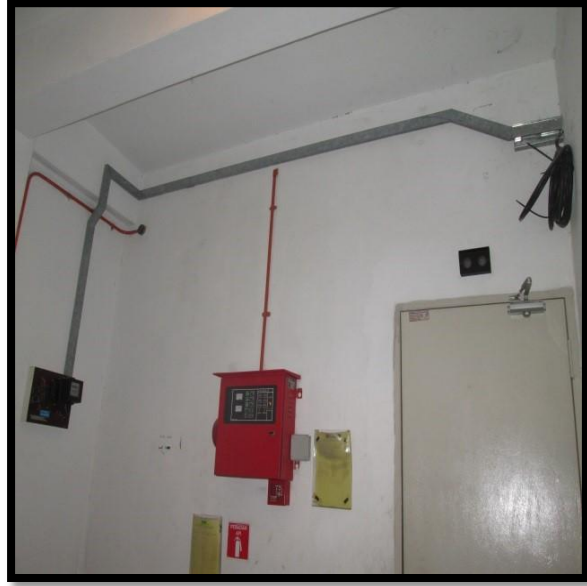
CABLE TRUNKING INSTALLATION
