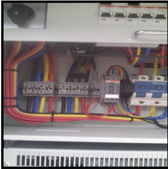
Installation T5 Cabinet TNB Incoming Termination
