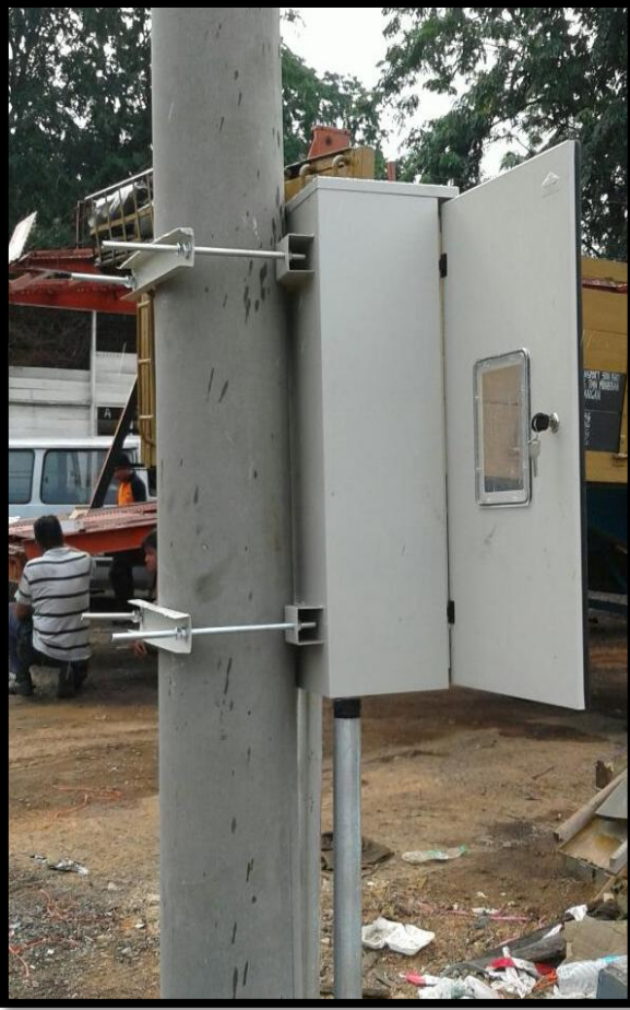
METER PANEL BOX INSTALLATION
