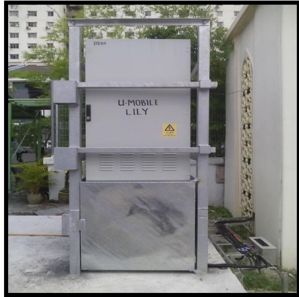
AFTER STEEL BELT INSTALLATION
