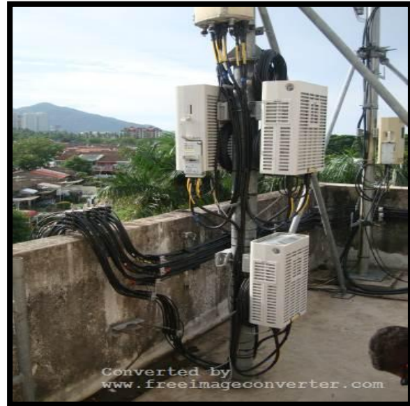
GABS HUAWEI RRU INSTALLTION
