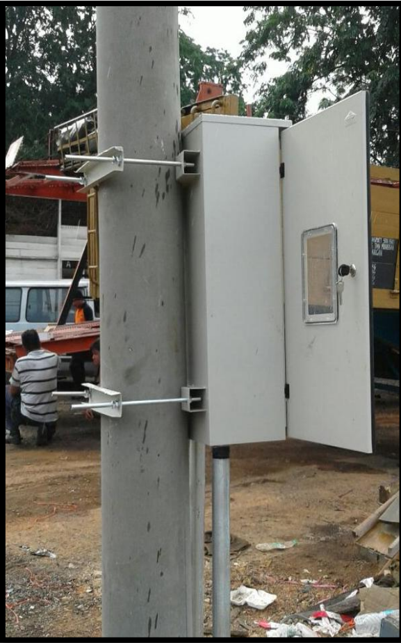
METER PANEL BOX INSTALLATION
