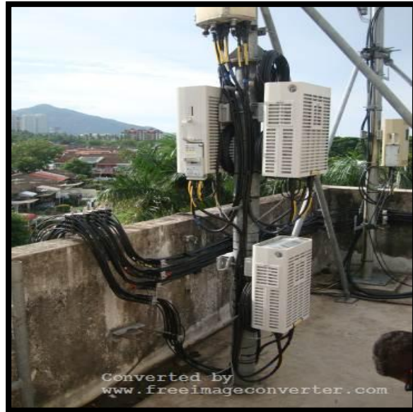
GABS HUAWEI RRU INSTALLTION
