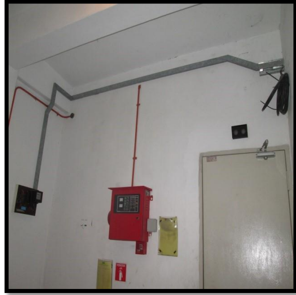
CABLE TRUNKING INSTALLATION
