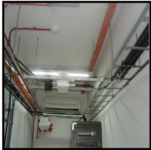
CABIN INTERNAL CABLE LADDER
