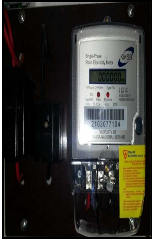
METER PANEL INSTALLATION
