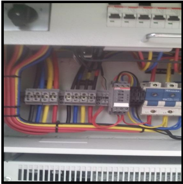
Installation T5 Cabinet TNB Incoming Termination
