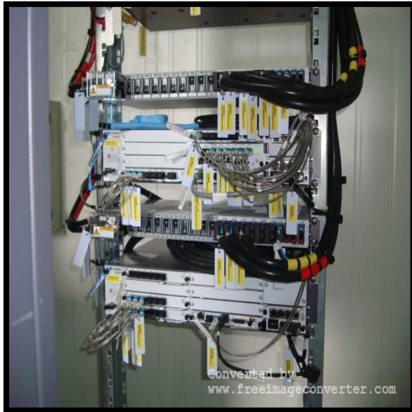
GABS HUAWEI BBU INSTALLATION
