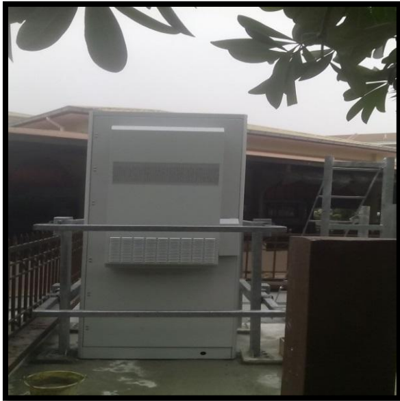
Installation T5 Cabinet C/W Lock Bar
