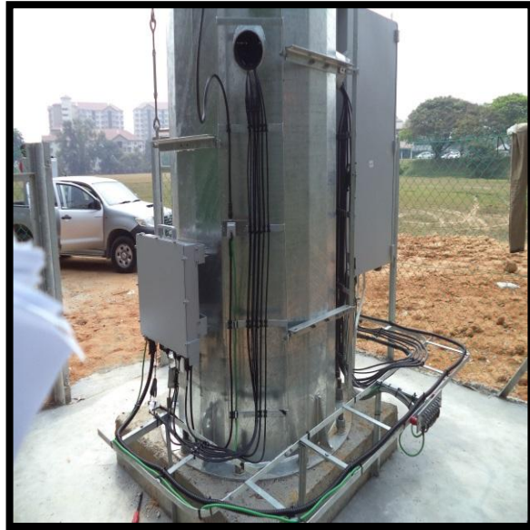
VERTICAL CABLE INSTALLATION
