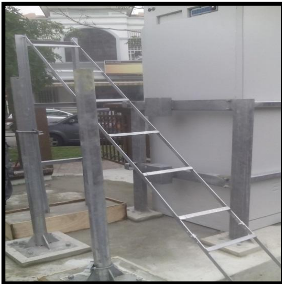
Installation Cable Ladder
